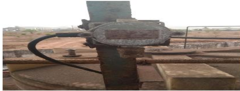
Annexure No.-11- Gas Detection System
