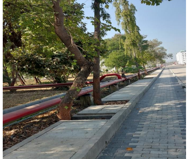
Storm Water Channel Diversion to save Ashok Tree
