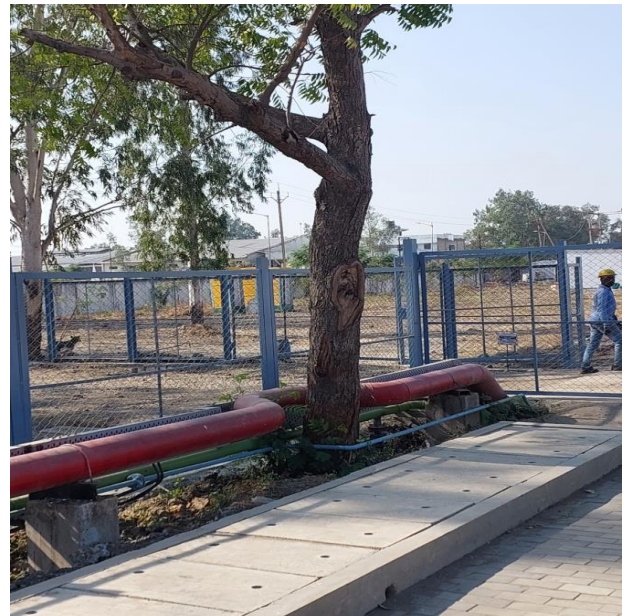
Hydrant Line Diversion to save Neem Tree
