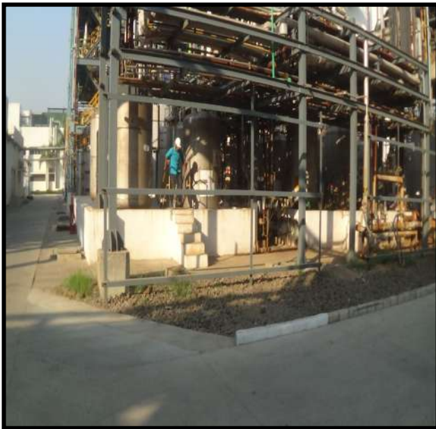
Fire observed by Mr. Ghanshyam Padhiyar at tank farm area
