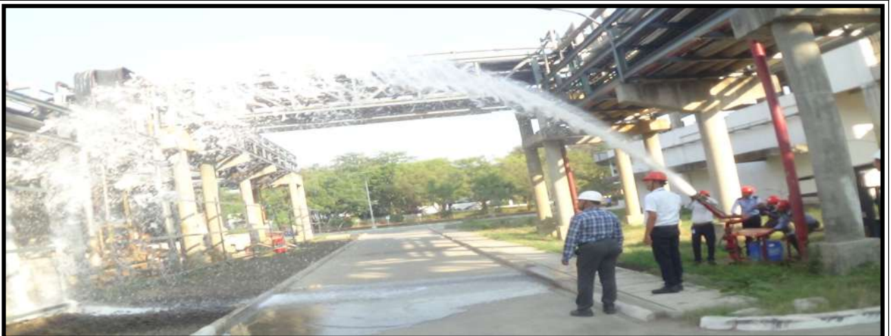
Starting fire fighting by the security and emergency team
