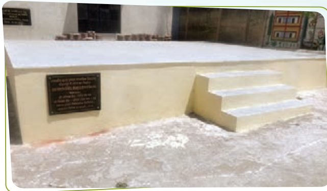
Construction of Platform
