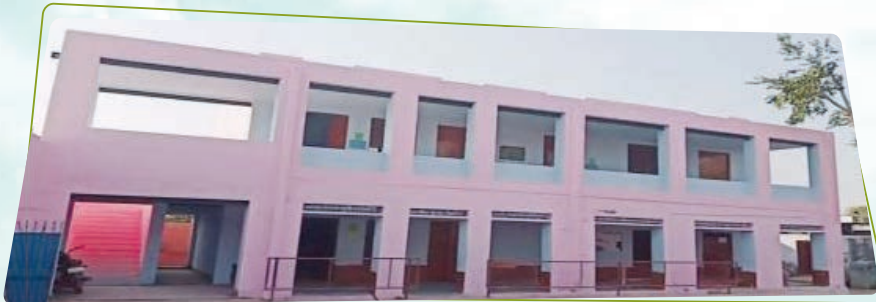
Hall Construction (30*20 ft)
